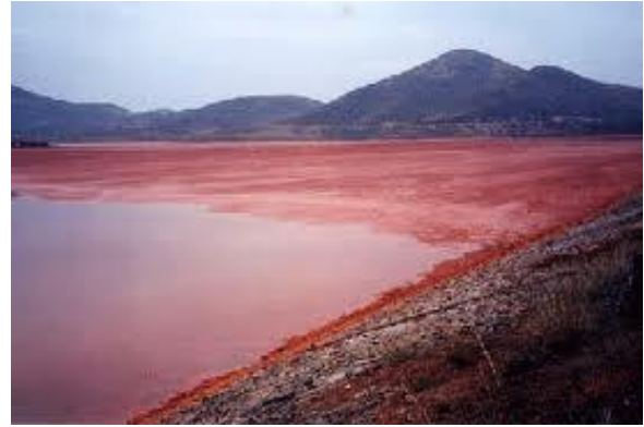
Figure 3. Lagooning red mud disposal (György & Tran 2010)
