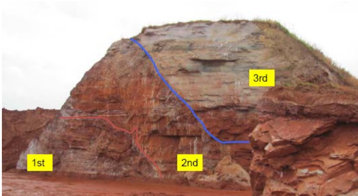
Fig. 4 Stages of building of the dam 8
