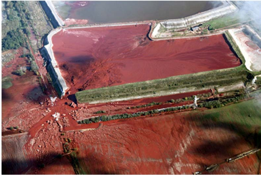
Fig. 9 Aerial photo of the Reservoir No. 10 after the dam failure in October 2010 25
